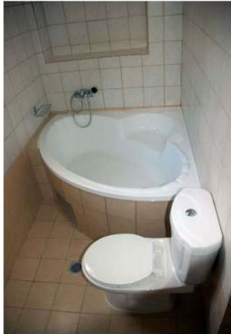
Newly fitted bathroom
