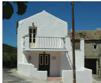
Front of property
