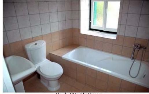
Newly fitted bathroom
