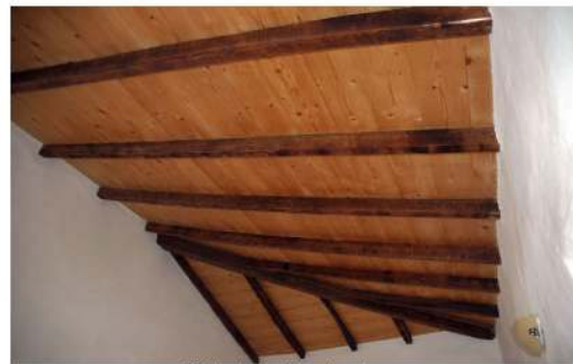
Cathedral ceiling in salon
